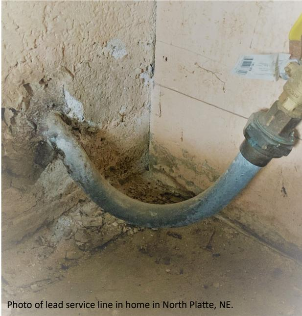
Photo of lead service line in home in North Platte, NE.
